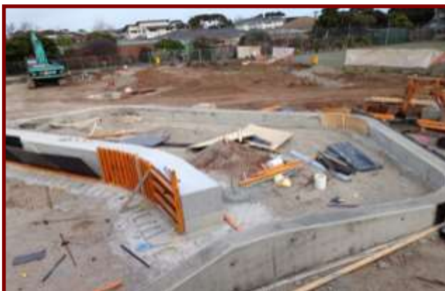
Niddrie Campus - The New Amphitheatre Under Construction
